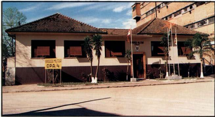
Fachada do Quartel – Montenegro
