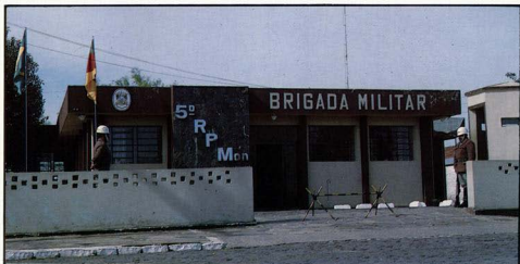
Fachada do Quartel – Santiago
