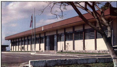
Fachada do Quartel – Montenegro
